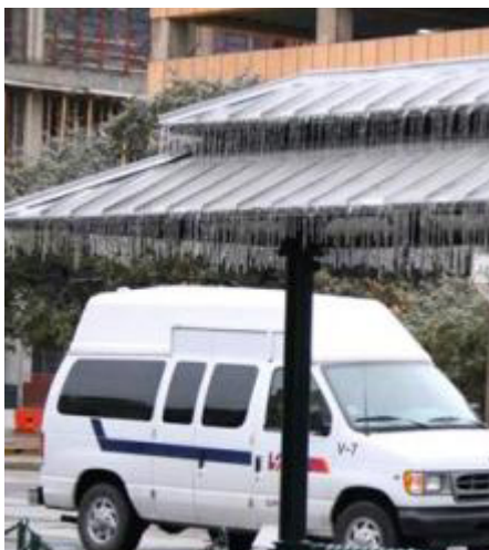
Thick ice coats downtown San Antonio, Texas, during a Jan. 2007 ice storm. (Photo courtesy of Kenneth E. Kehoe)
