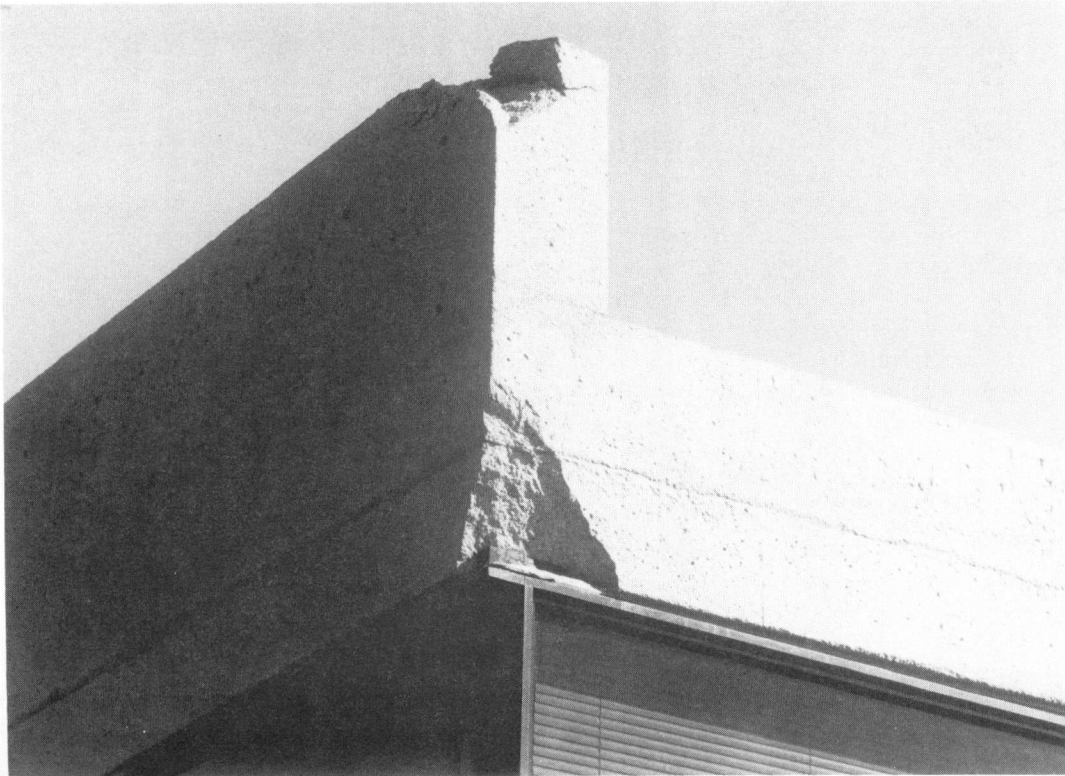
Inspiration strikes often on the mesa, but it was lightning that crumbled a chunk of the A tower's southwest corner in July 1978. Project 2000 will spruce up the outside of the Mesa Lab and update the inside. (Photo by Bob Bumpas.)
