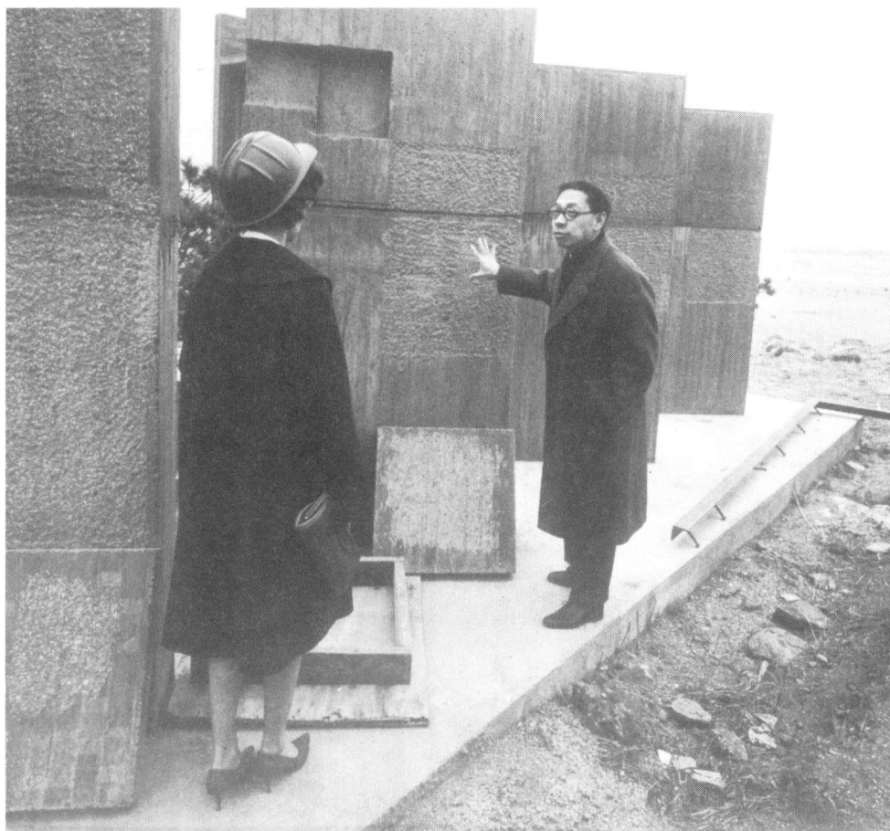
I.M. Pei (right) experimented with several finishes to the concrete used on the Mesa Lab. Some of the possibilities were on display early in construction.
