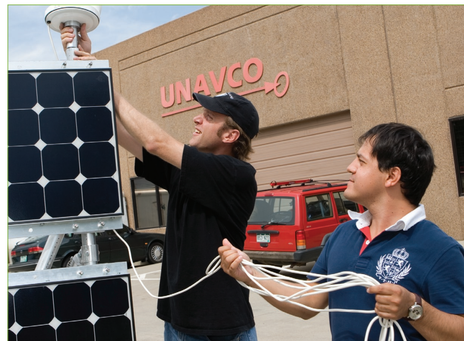
Ezer Patlan with UNAVCO polar engineer and project mentor Seth White working on a polar remote power and communication system
